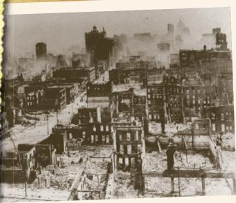
The shifting of the earth during the quake caused underground pipes to rupture. Some of those pipes carried natural gas, a highly flammable fuel. The leaking gas caused fires. Other broken pipes were water mains—and when the mains broke, that meant that firefighters had no water to use to fight the fires. Unchecked, the fires spread quickly.
