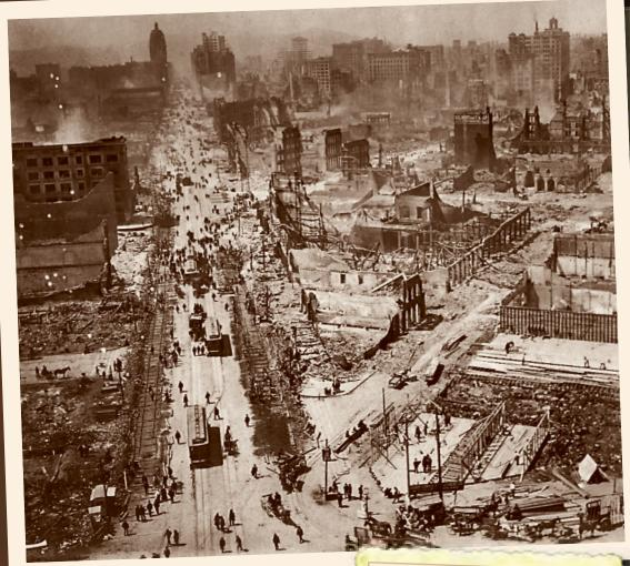
Many parts of the city were built on former marshes that had been filled in with sand and other debris. This "made land" was very unstable and turned to mush during the earthquake—something called liquefaction. The soft, soggy ground could no longer support the buildings and many of them simply collapsed.
